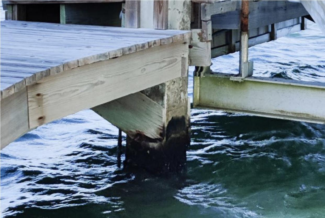
**Figure 25:** Tidal fluctuation at adjacent dock indicated by darkened area.
