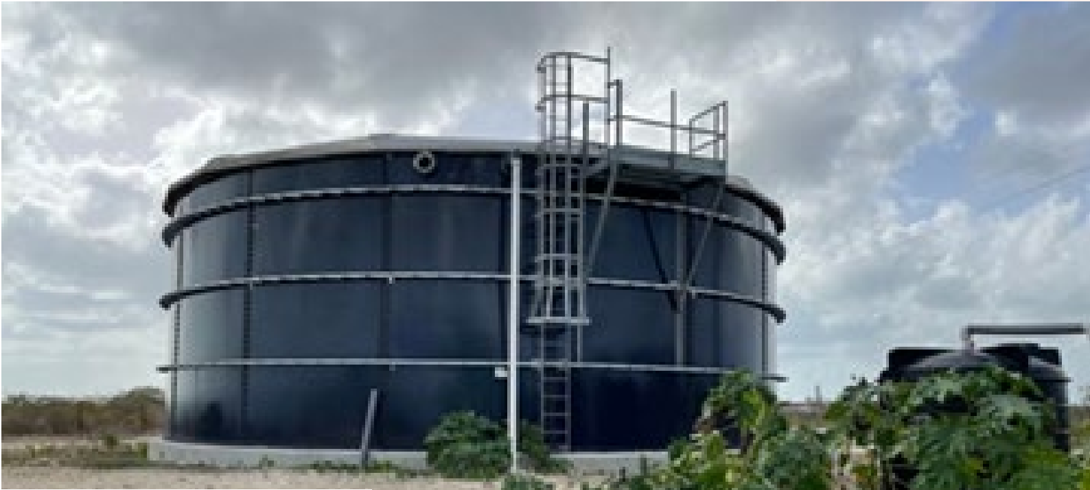
APUA River Reverse Osmosis Water Storage Tank for treated water Source: Future Barbuda
