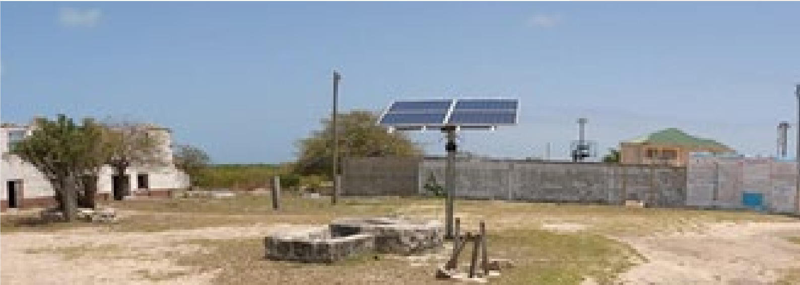
Water well with solar pump, Codrington Source: Future Barbuda
