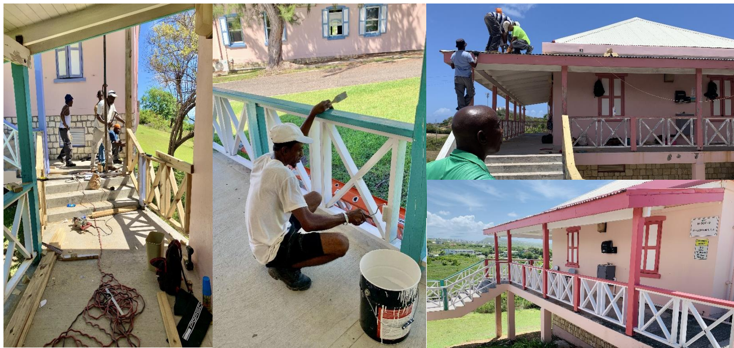
PUBLIC WORKS DEPARTMENT AT WORK
